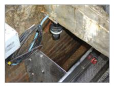
dB3 WITH DRIP SHIELD MOUNTED IN CSO CHAMBER
