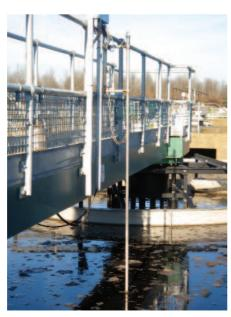
VIPER TRANSDUCER ON CONDUIT WITH ROTATING BRIDGE
